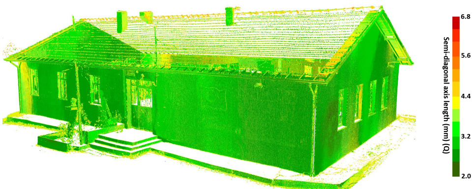
FIGURE 17 Visualisation of the Q values of the school building point cloud after the incidence angle-based decimation step with t_\gamma = 60^\circ .
