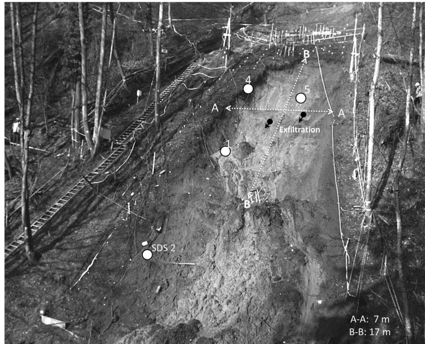
Fig. 7 Post event record of the landslide and relative location of the soil deformation sensors with respect to the destabilised soil mass
